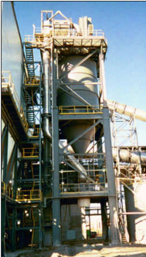
DustMASTER 200 tph Series I system installed under storage silo with truck drive through.
