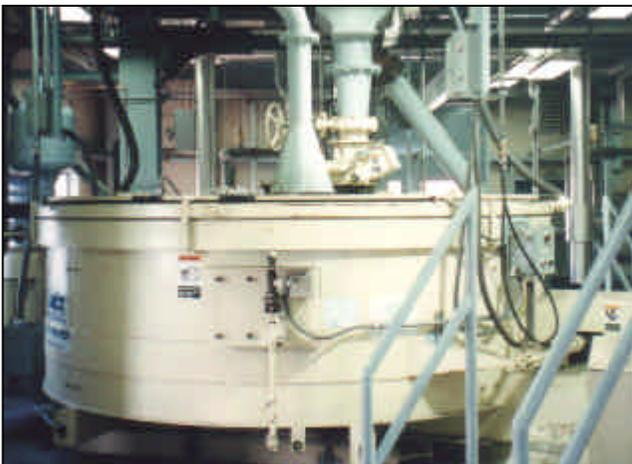
The 40 tph DustMASTER unit in place under an economizer ash silo.
