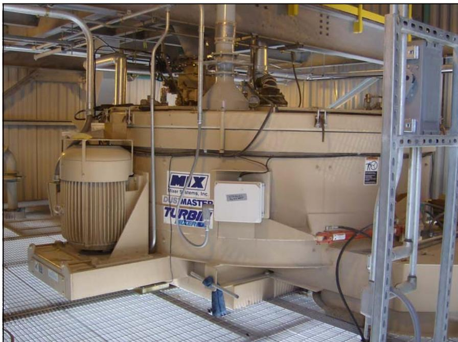
DustMASTER 40 TPH Series II system installed under storage silo.
