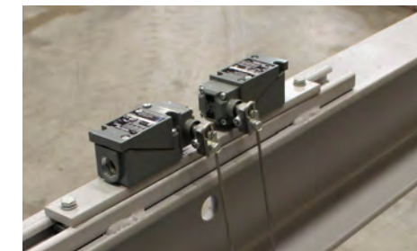
Bucket position limit switches are adjustable
